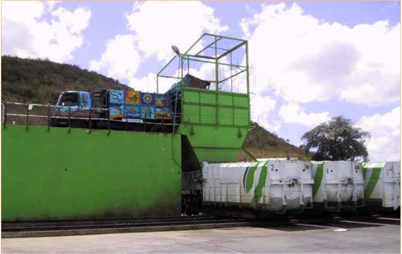
FIGURE 2-3 Outdoor Transfer Station with compaction of waste
